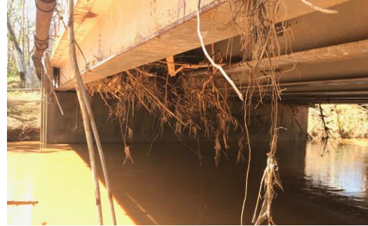
Figure 9 Bridge No. 55 Inspection Photo Post-Maria [14]
