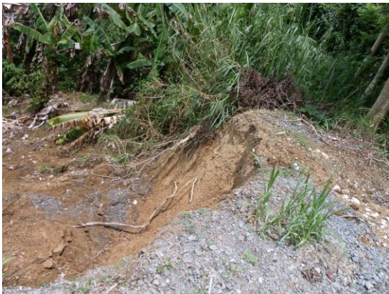
Figure 4 Slope Side-view of the Failure Surface
