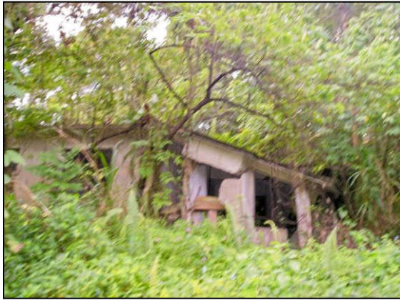
Figure 2 Piedras Blancas Landslide: Abandon residence
