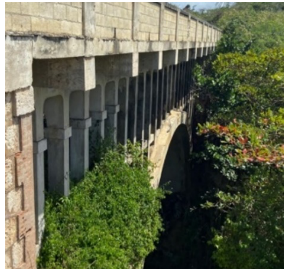
Figure 7 View of south side of the bridge
