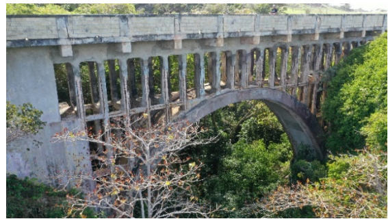
Figure 4 Bridge in its present condition
