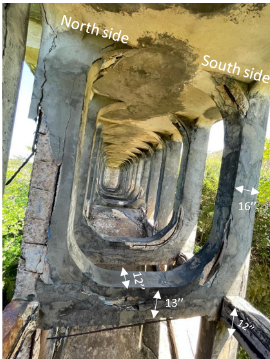
Figure 5 Interior of bridge
