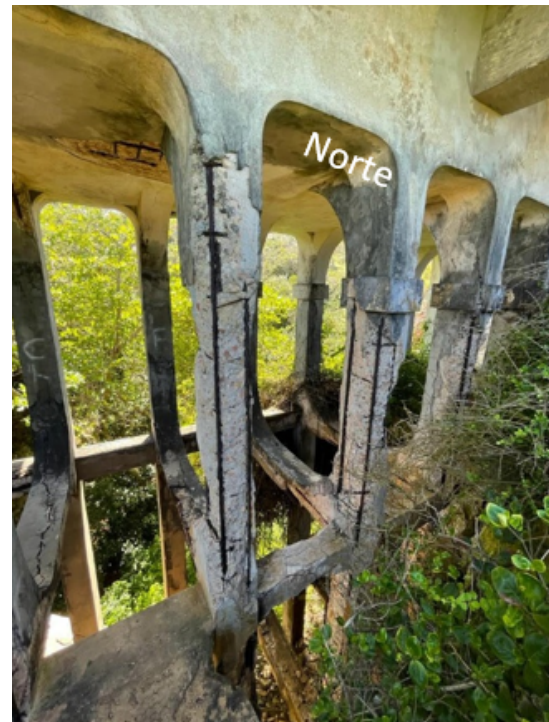
Figure 6 View of north side of the bridge
