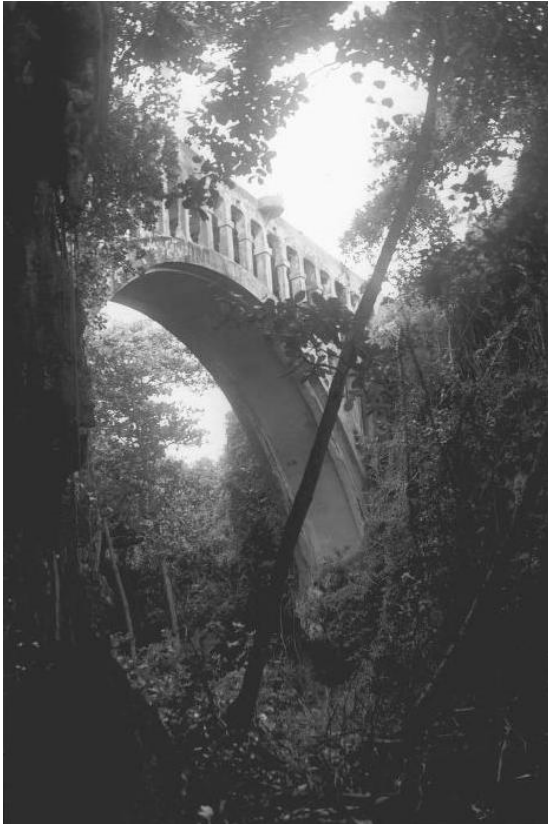
Figure 2 Original condition of the bridge
