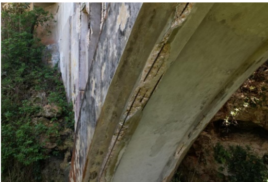
Figure 9 The inferior side of the arch
