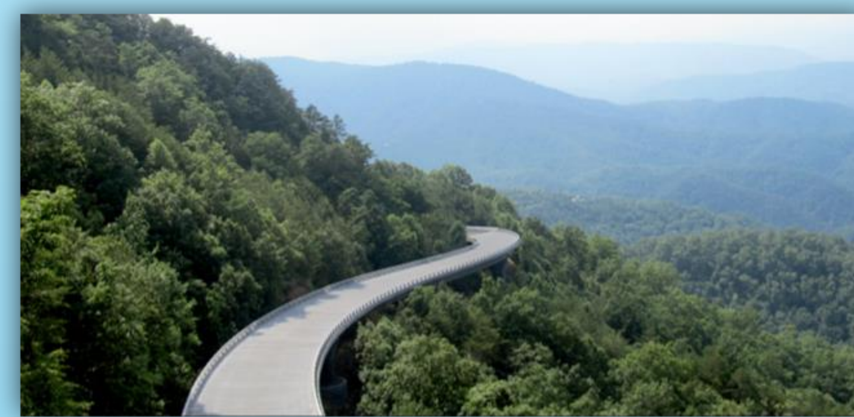
Foothills Parkway Bridge 2 - Project EFLHD completed for the National Park Service Image retrieved from reference [2]
