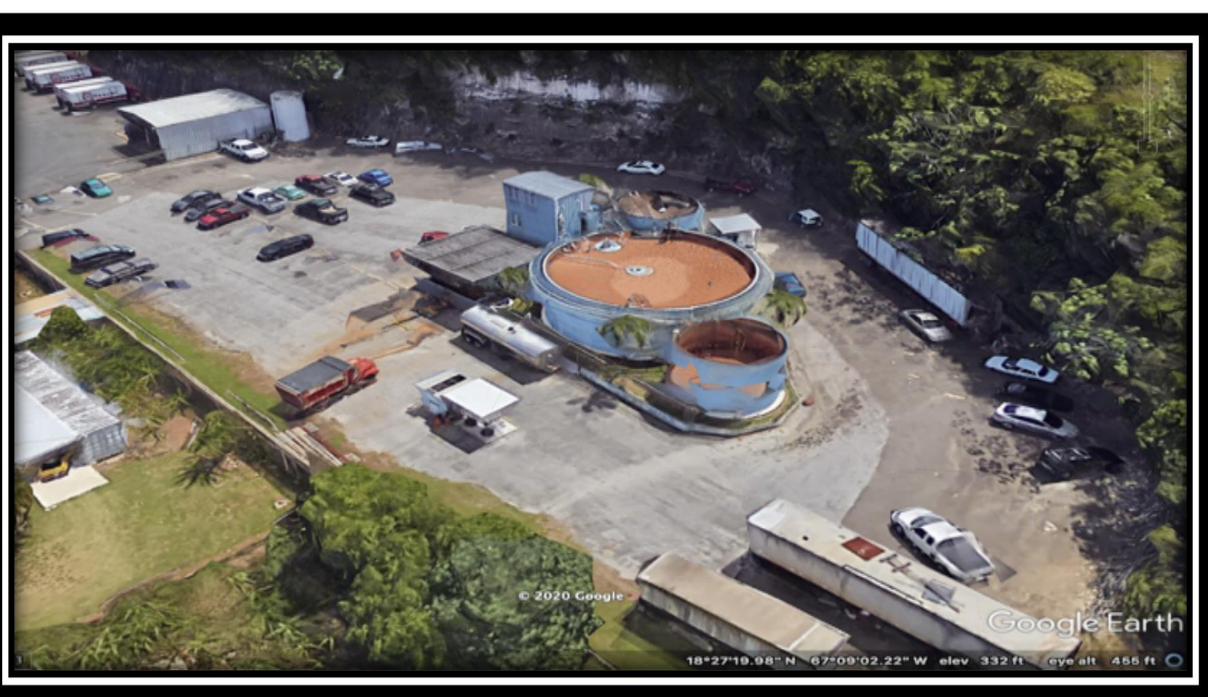
Figure 2 Before "Vida" Plant Expansion Water Treatment Plant
