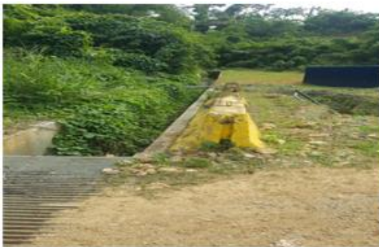
Figure 13 Toa Baja Municipal Solid Waste Landfill Concrete Channel from the Community’s Natural Sinks to “El Hoyo de Minga” Sink (February 2019)
