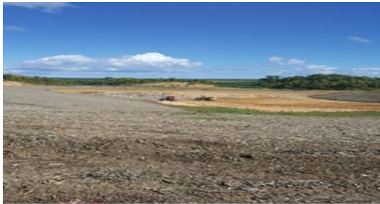
Figure 3 Actual Solid Waste Site Deposit at Carolina Municipal Landfill (January 2019)
