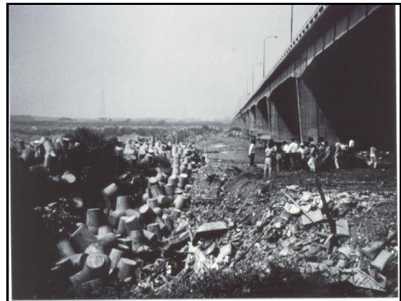
Figure 9 Channel Response to In-stream Gravel Removal [4]
