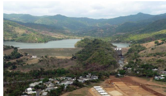
Figure 1 Patillas Dam, Reservoir and Spillway [2]
