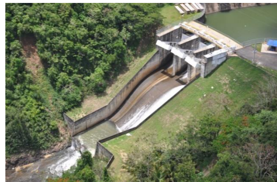
Figure 3 An Aerial View of the Spillway for Lago Patillas
