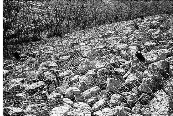
Figure 6 Wire Enclosed Riprap
