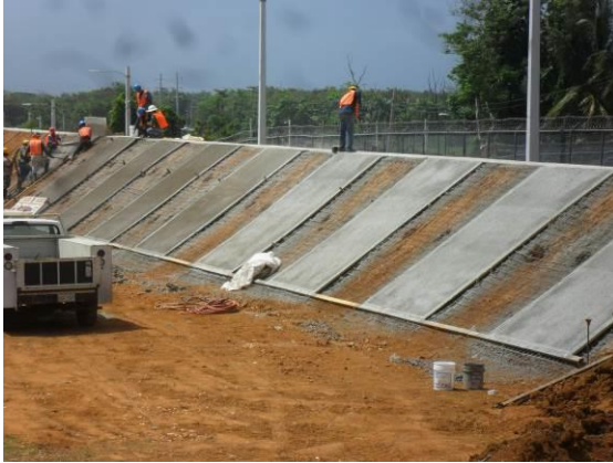
Figure 1 Shotcrete Dike Liner under Construction
