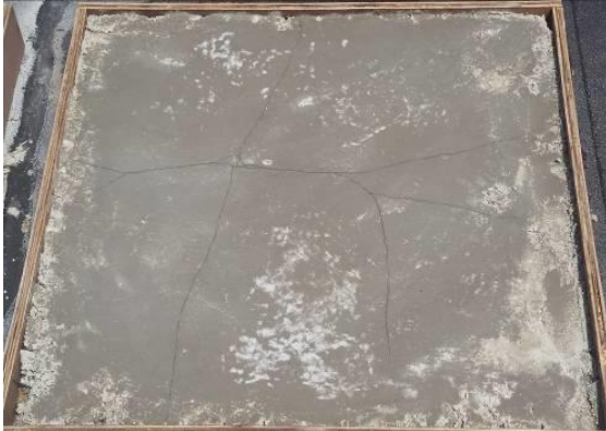
Figure 7 Fly Ash Batch Cracking Pattern
