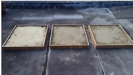
Figure 2 Shotcrete Batches on the Roof
