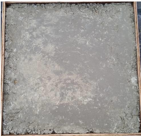
Figure 8 Fiber Reinforced Batch Cracking Pattern
