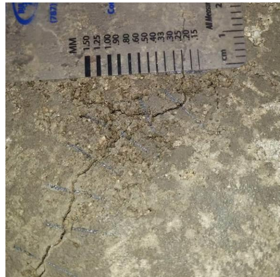
Figure 5 Measuring Cracks with a Gauge
