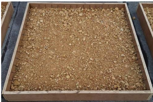
Figure 4 Clay Base Installed
