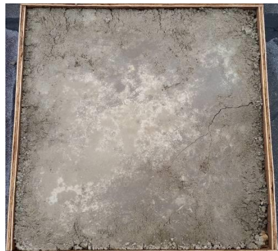
Figure 6 Control Batch Cracking Pattern
