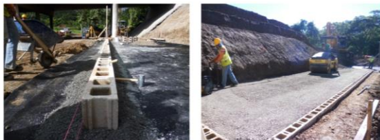
Figure 6 Abutment and Wing Walls (CMU) GRS
