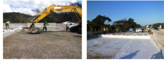
Figure 7 Integrated Approach Zone (IBS)
