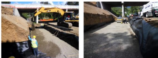
Figure 5 Reinforced Soil Foundation
