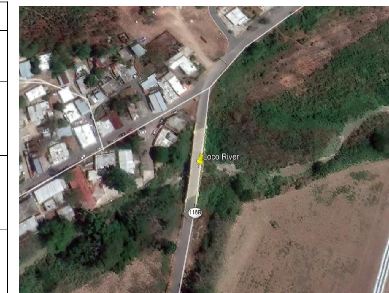
Figure 3: Geolocation of Loco River Bridge (Google Earth, 2020)
