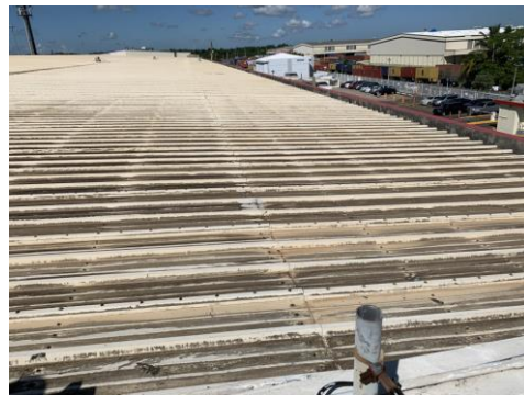
Figure 3 Building Roof Condition
