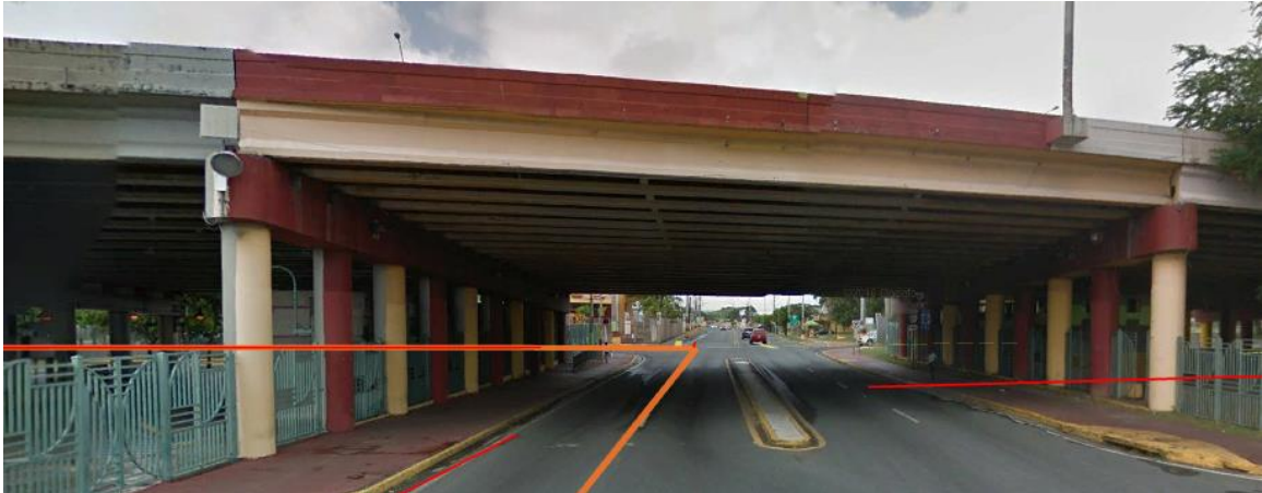
Figure 6-204 Bridge on the Evacuation Route of Francisco Oller School (Google Earth – 2016)
