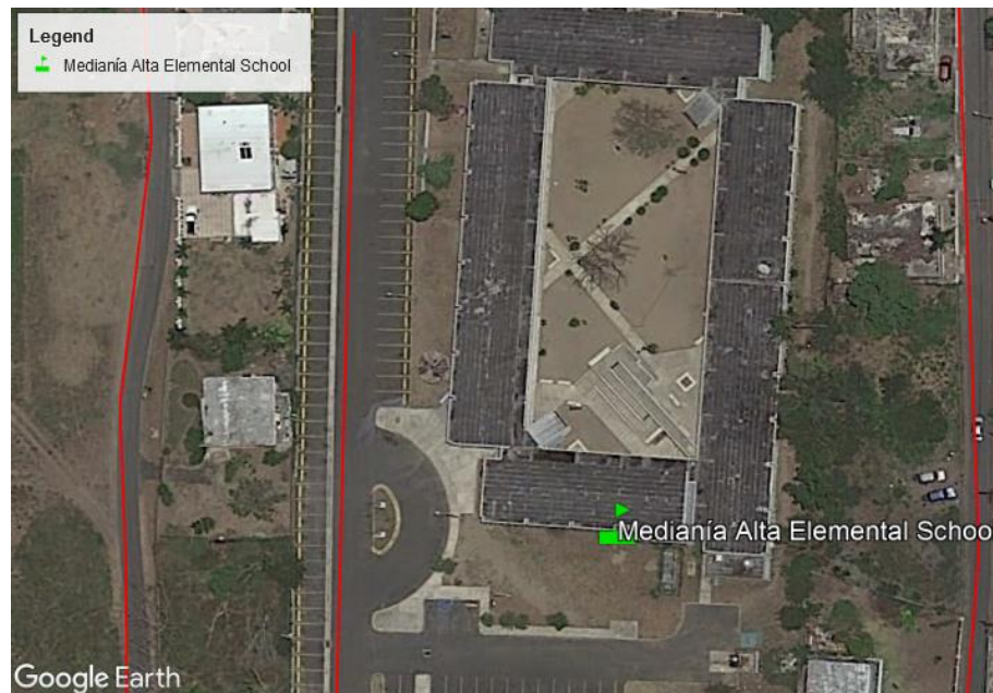
Figure 7-1 Medianía Alta Elemental School (Google Earth – 2018)
