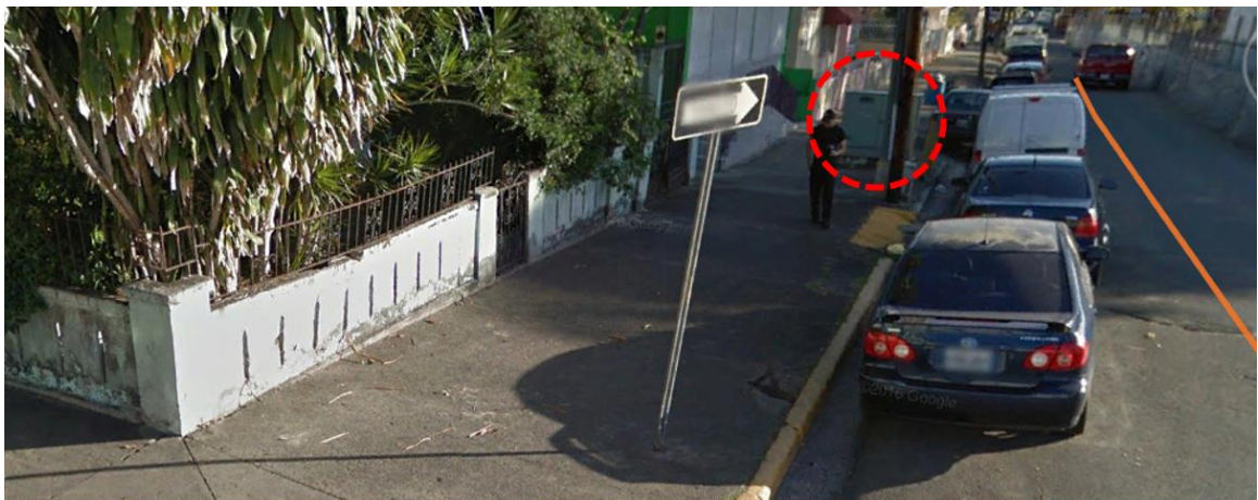
Figure 6-327 Sidewalk on Felipe R. Goyco Street from the Evacuation Route of Luis Llorens Torres School in Street View (Google Earth – 2016)
