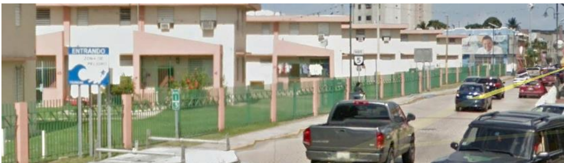
Figure 6-185 Entering Hazard Zone Sign Near the Perimeter of Francisco Oller School (Goole Earth – 2016)
