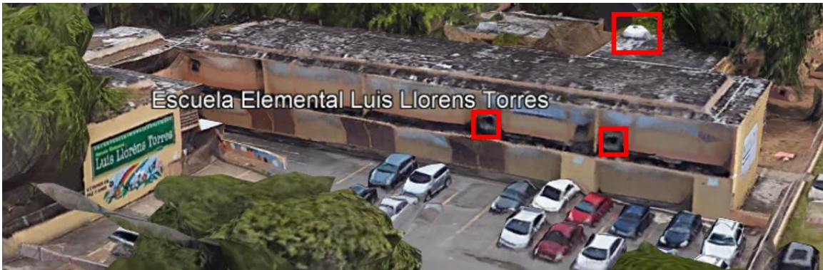
Figure 6-262 Nonstructural Falling Hazards at Luis Llorens Torres School (Google Earth – 2016)
