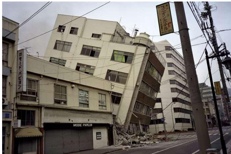
Figure 2-5 Building collapse in the earthquake of 1995 in Kobe, Japan
