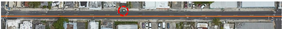
Figure 6-308 Fourth Section of Sidewalk on Pellín Rodríguez Street from the Evacuation Route of Luis Llorens Torres School in Plan View (Google Earth – 2016)
