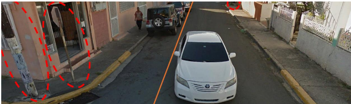
Figure 6-324 First Section of Sidewalk on Catalino “Tite” Curet Alonso Avenue from the Evacuation Route of Luis Llorens Torres School in Street View (Google Earth – 2016)
