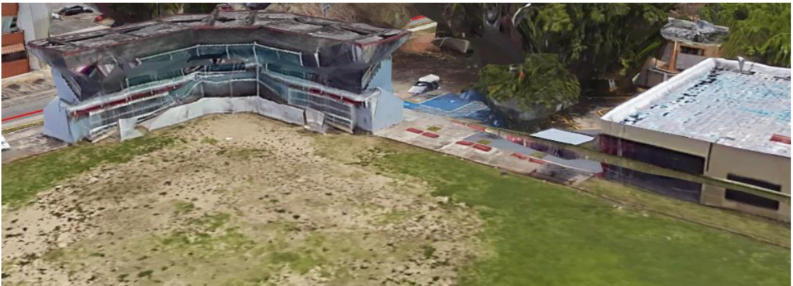
Figure 6-260 Cancha (Llorens) Monserrate Kike Ríos as Adjacent Building to Luis Llorens Torres School (Google Earth – 2016)
