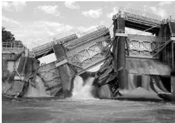
Figure 2-8 Collapse of the Shih-Kang dam
