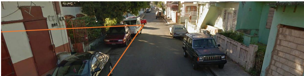
Figure 6-325 Second Section of Sidewalk on Catalino “Tite” Curet Alonso Avenue from the Evacuation Route of Luis Llorens Torres School in Street View (Google Earth – 2016)
