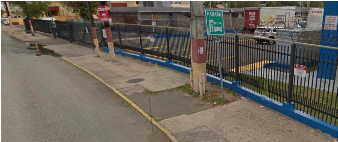
Figure 6-224 Poles in Fourth Section of Sidewalk on Las Nereidas Avenue from the Evacuation Route of Francisco Oller School in Street View (Google Earth – 2016)
