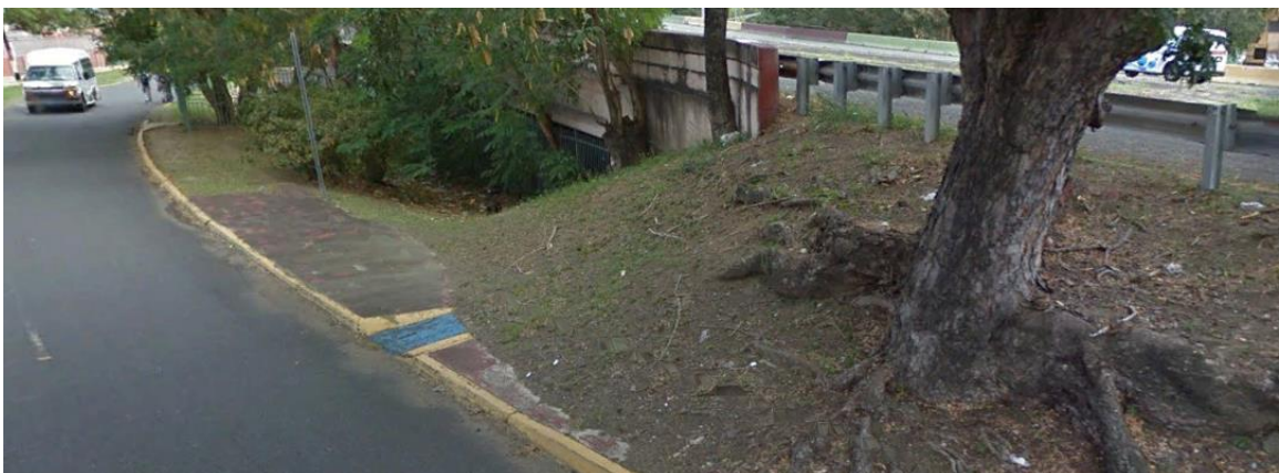
Figure 6-238 Incomplete Sidewalk on El Caño Avenue from the Evacuation Route of Francisco Oller School in Plan View (Google Earth – 2016)
