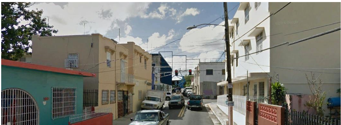
Figure 6-277 Power Lines on the Evacuation Route of Luis Llorens Torres School through Pellín Rodríguez Street [End of the Street] (Google Earth – 2016)
