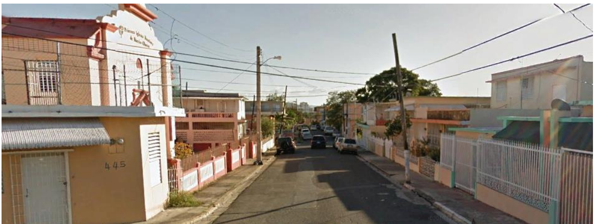
Figure 6-280 Power Lines on the Evacuation Route of Luis Llorens Torres School through Lippit Street (Google Earth – 2016)
