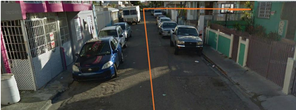
Figure 6-316 Poles in Sidewalk on Los Santos Street from the Evacuation Route of Luis Llorens Torres School in Street View (Google Earth – 2016)
