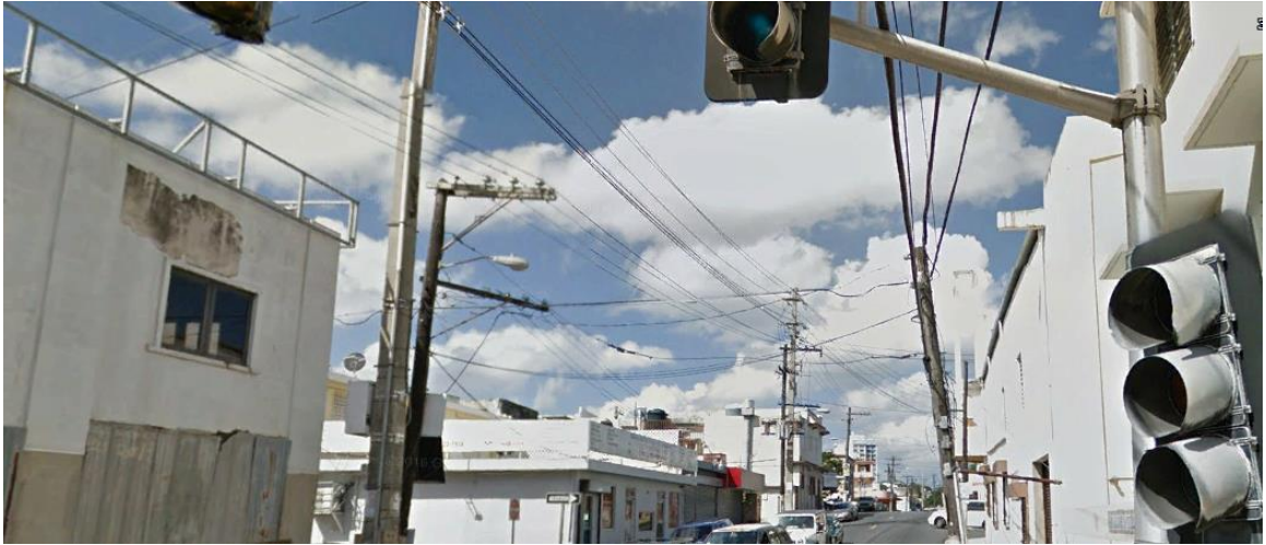
Figure 6-279 Power Lines on the Evacuation Route of Luis Llorens Torres School through Eduardo Conde Avenue (Google Earth – 2016)
