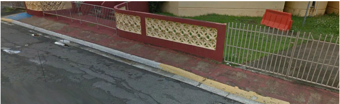
Figure 6-228 Sidewalk on Olivo Street from the Evacuation Route of Francisco Oller School in Street View (Google Earth – 2016)
