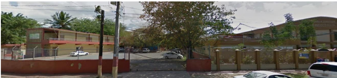
Figure 6-177 Onofre Carballeira School Adjacent to Francisco Oller School (Google Earth – 2016)
