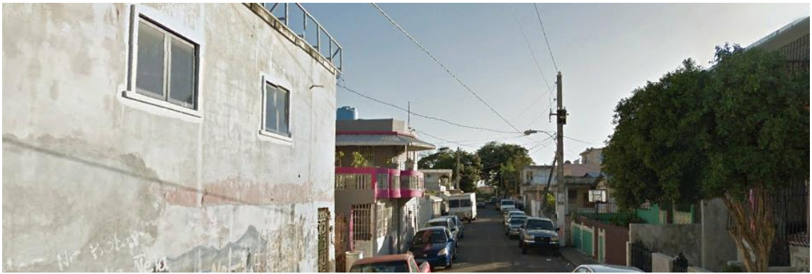
Figure 6-278 Power Lines on the Evacuation Route of Luis Llorens Torres School through Los Santos Street (Google Earth – 2016)
