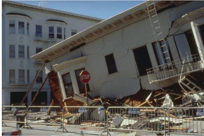
Figure 2-9 Landfill liquefied in the 1989 Loma Prieta earthquake.
