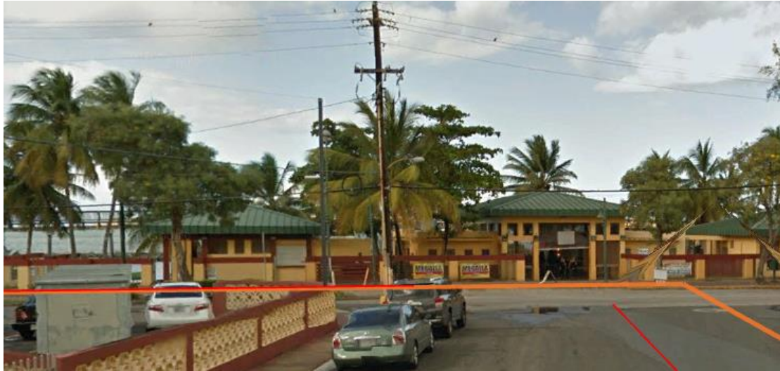
Figure 6-200 Power Lines on the Evacuation Route of Francisco Oller School through Olivo Street (Google Earth – 2016)
