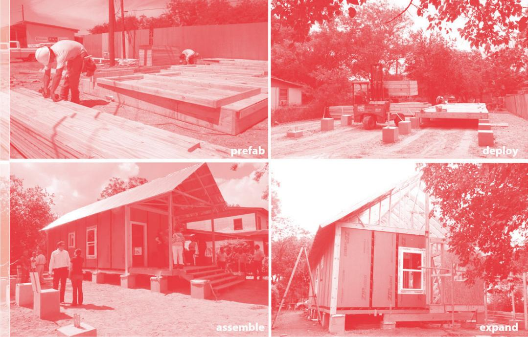
Figure 6. RAPIDO construction process.
