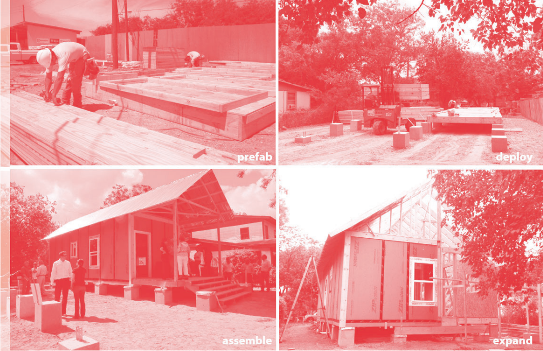
Figure 6. RAPIDO construction process.
