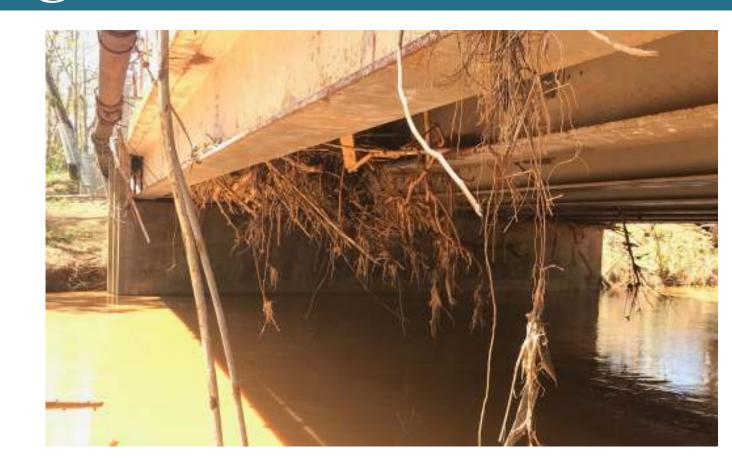
On October 4, 2017, Bridge No. 55 was inspected for damage after Hurricane Maria. Inspection findings included debris accumulation and moderate erosion at the river banks. However, after inspecting for scour at abutments by means of wading, no scour was found, therefore the inspected scour Post-Maria was determined to be 0.00 m [9].
