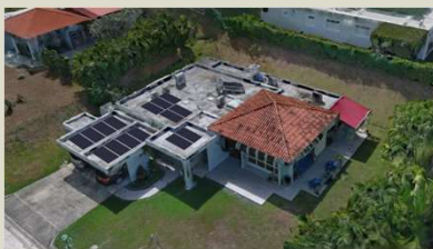
3D Scanning of the residential Building showing the PV system (Source: Verdicta PSC)
