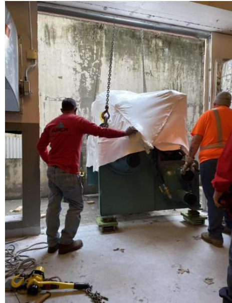
Figure 5 Getting the new chiller into the basement
