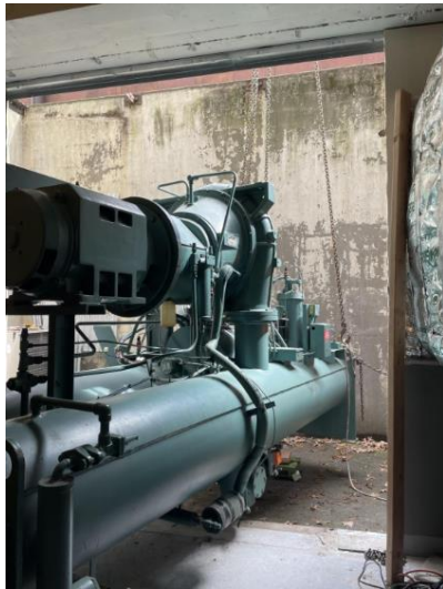
Figure 3 Removal of the old chiller from the basement
