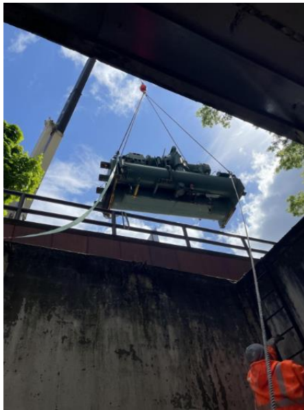
Figure 4 Removal of the old chiller from the basement II
