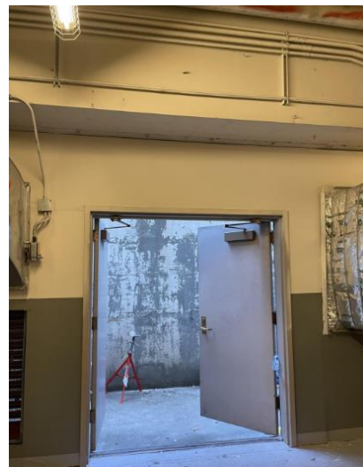
Figure 6 Reconstruction of the demolished frame and wall
