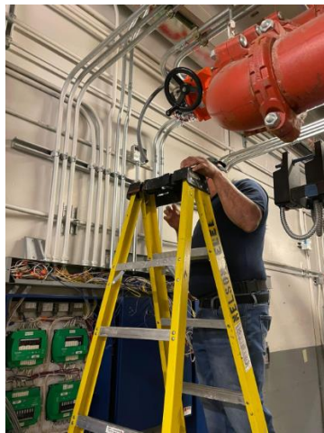
Figure 7 New Communication Cable Installation
