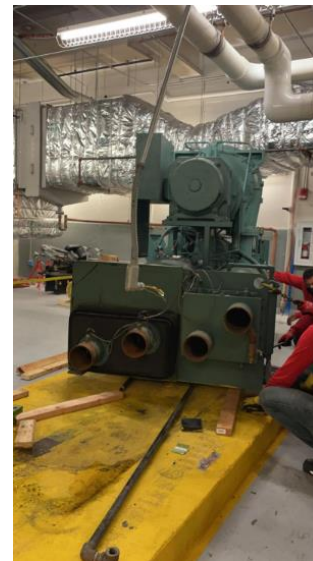
Figure 2 Second day onsite work
