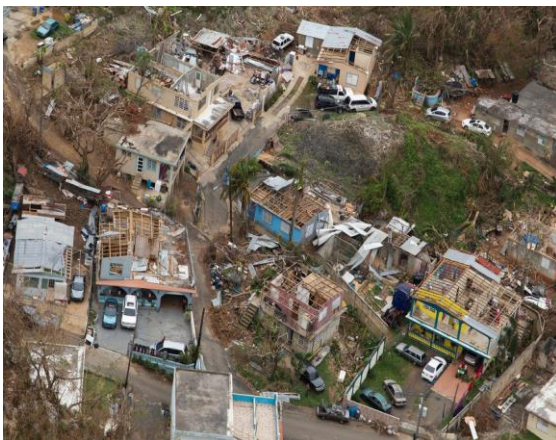
Figure 2 A neighborhood in Puerto Rico where Several Houses Lost All Their Roofs (Source: FEMA)
