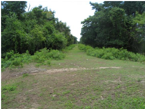
Figure 4 Downstream view of Right Side Levee of Rio Humacao from Bridge on State Road PR-53
