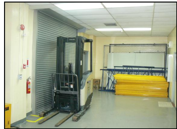
Figure 4 Main Corridor (West View)
