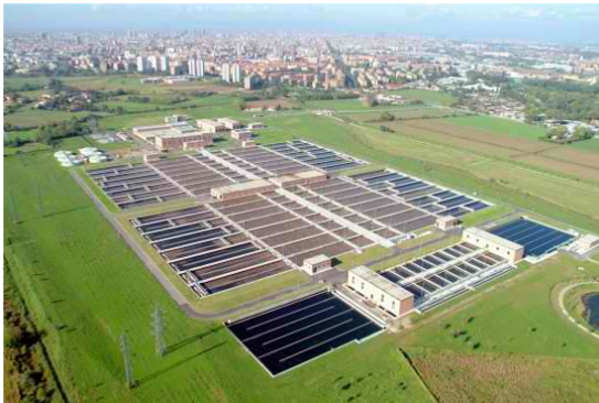
Figure 1 Nosedo WWTP, Milan Italy
