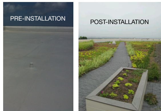
Figure 7 Overview of Pre and Post Condition (Ballaja Green Roof Installation)
