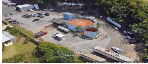
Figure 1 Before “Vida” Plant Expansion Water Treatment Plant
