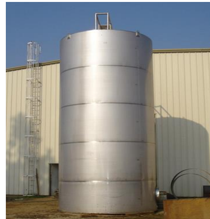
Figure 6 Storage Tank Replacement
