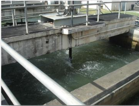
Figure 1 Aeration Oscillation Mechanism
