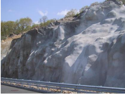
Figure 7 Shotcrete Facing Over Rock Slope Example
