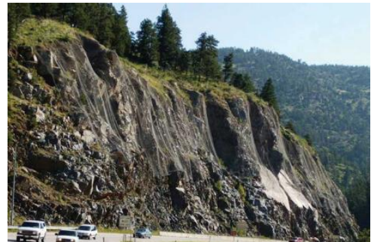
Figure 9 Drape Mesh Facing Over Rock Slope Example
