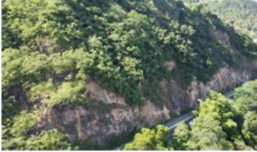
Figure 2 Aerial View of Rock Slope
