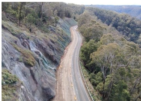
Figure 5 Wire Mesh Facing Over Rock Slope Example
