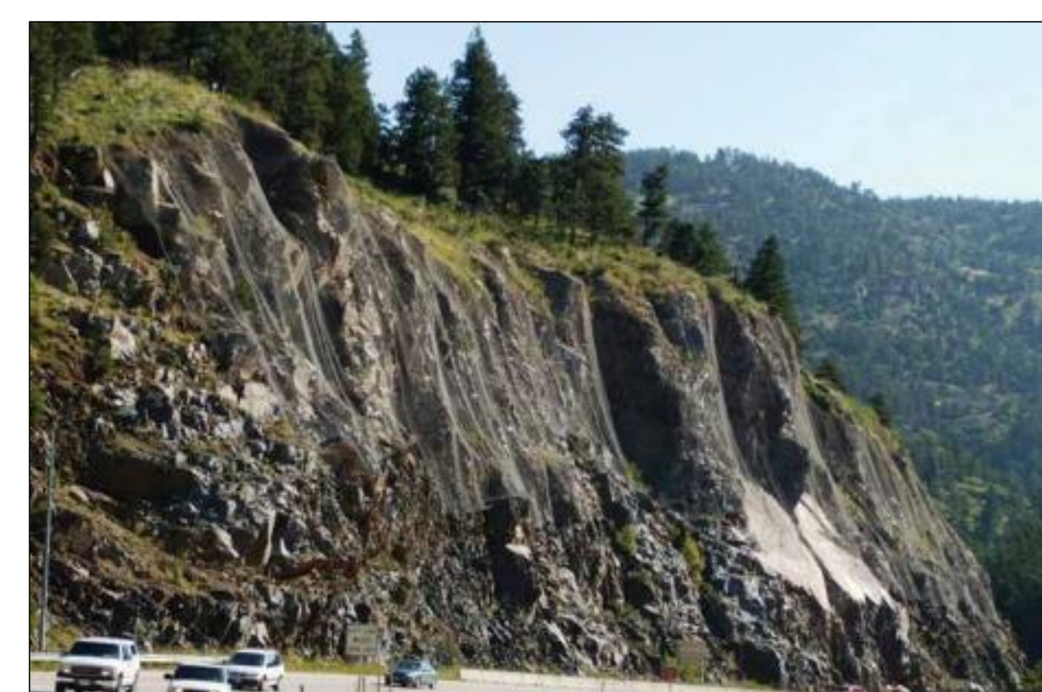
Drape Mesh Over Rock Slope Example
