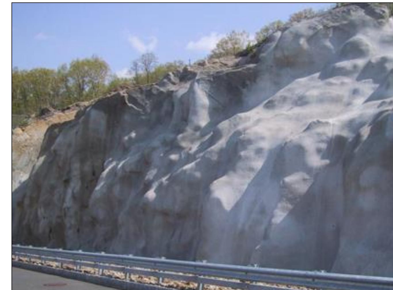
Shotcrete Facing Over Rock Slope Example
