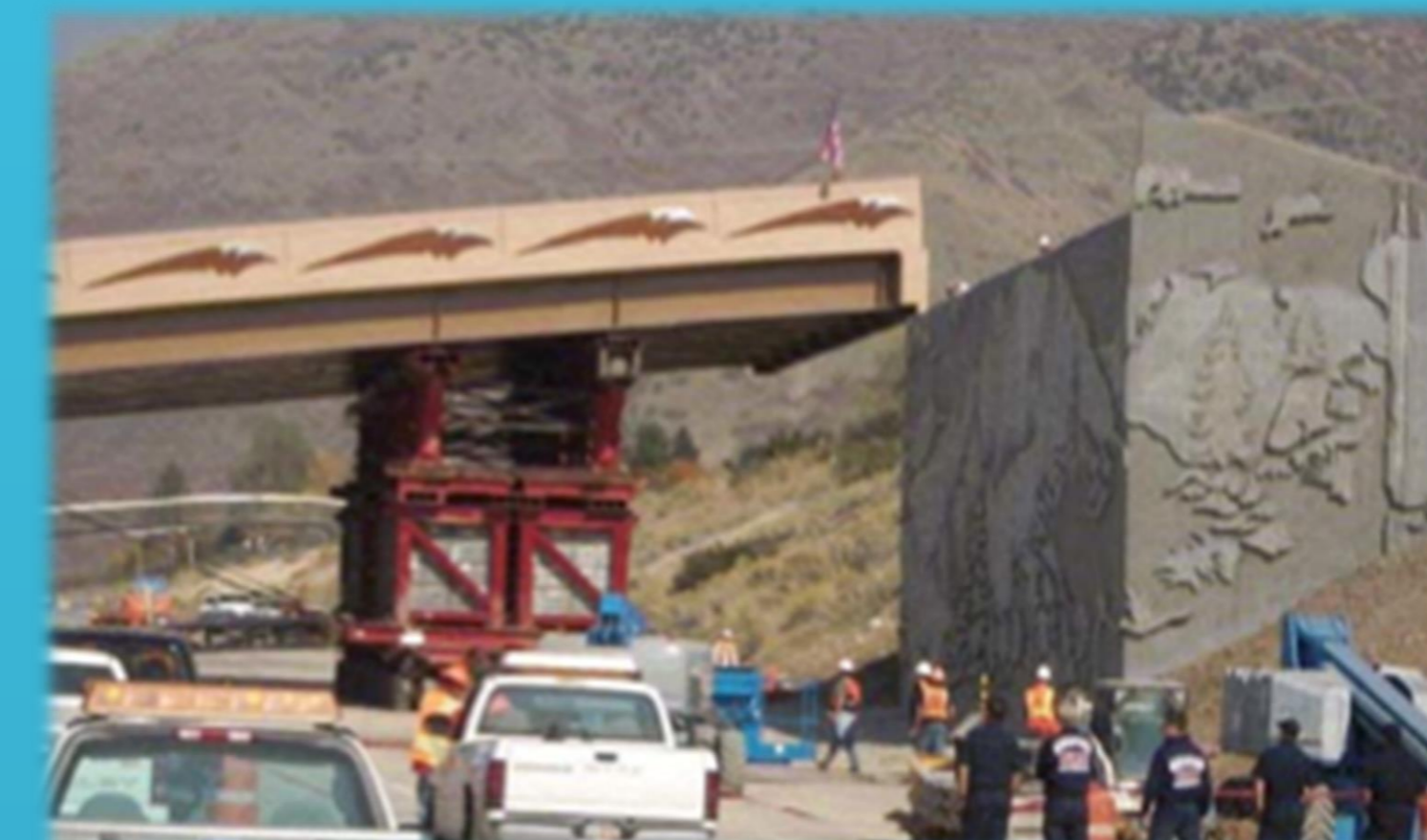
The Figure 2: Self-propelled modular transporter (SPTs). [3]
