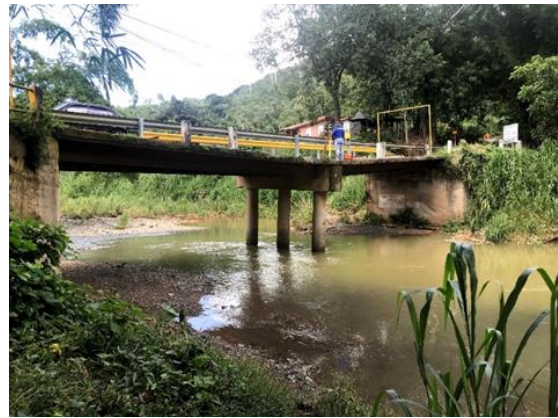
Figure 1 Analyzed Bridge Structure
