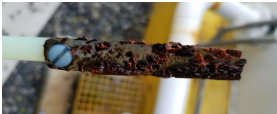
Figure 7 Mild Steel Corrosion Coupon after 60 Days Exposed to Chlorinated Water
