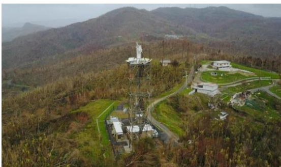
Figure 4 WSR-88D Radar after its Destruction
