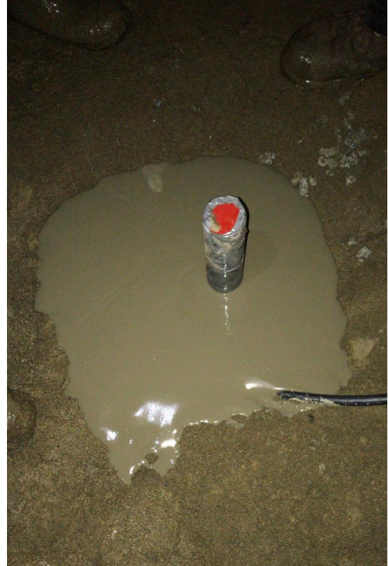
Figure 11 Finished Micropile
