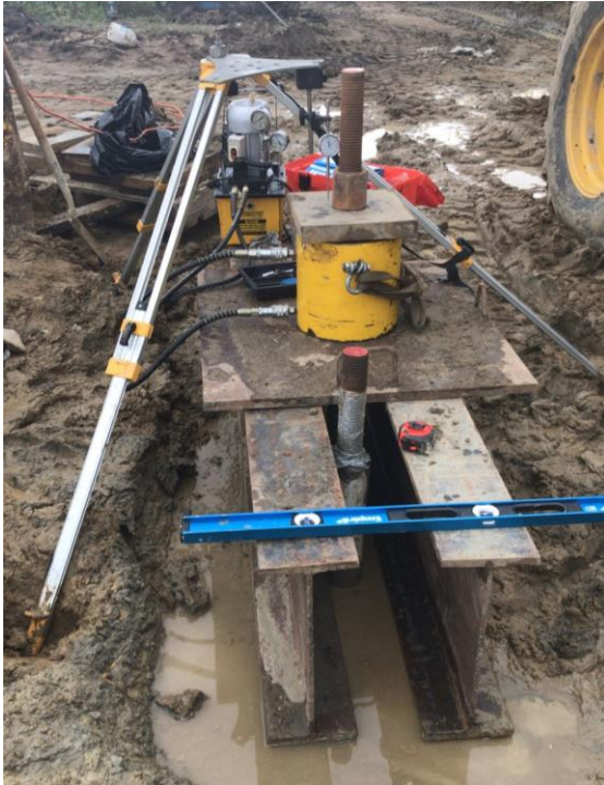
Figure 12 Load Test Set-Up
