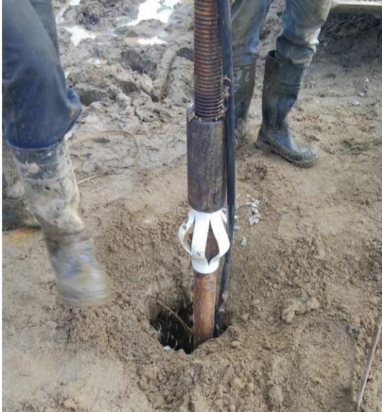
Figure 9 Micropile Reinforcing Bar Installation
