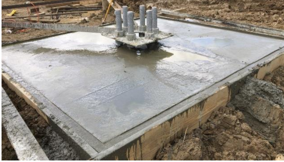
Figure 15 Picture Showing Completed Pile Cap
