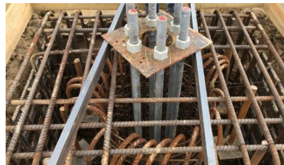
Figure 14 Picture Showing Steel Reinforcement Partially Completed
