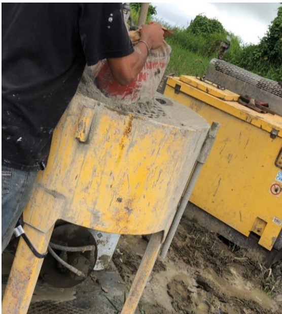
Figure 10 5,000 psi Neat Cement Grout Mixing and Pumping
