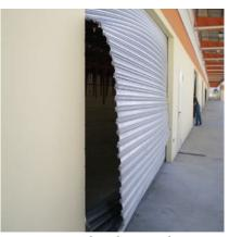
Figure 10 - Windward Doors Blown-Out
