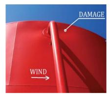
Figure 9 - Damaged Water Tank Riser
