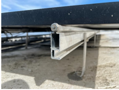
Figure 6 Long Leg and Rail of Mounting System H
