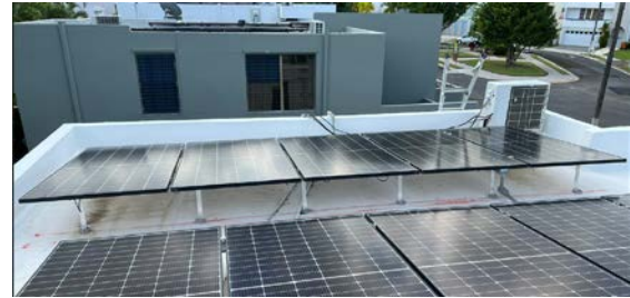
Figure 8 Mounting System H with N+1=L Installation Pattern
