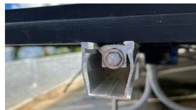
Figure 5 Mounting System U Rail Shape
