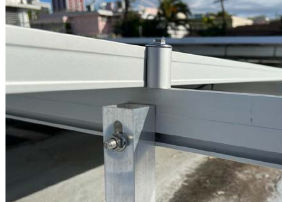
Figure 10 Mounting System B Long Leg Aligned with Clamp
