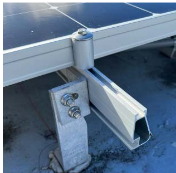
Figure 3 Short Leg and Rail of Mounting System B
