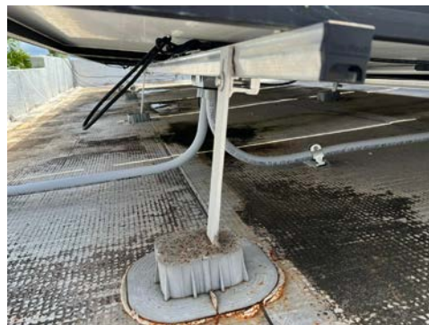
Figure 4 Long Leg of Mounting System U
