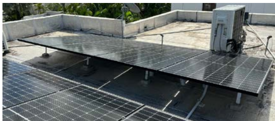
Figure 7 Mount System U with N=L Installation Pattern
