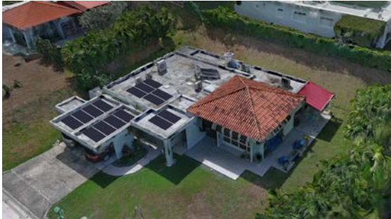
Figure 1 3D Scanning of Residential Building (Source: Verdifica PSC)
