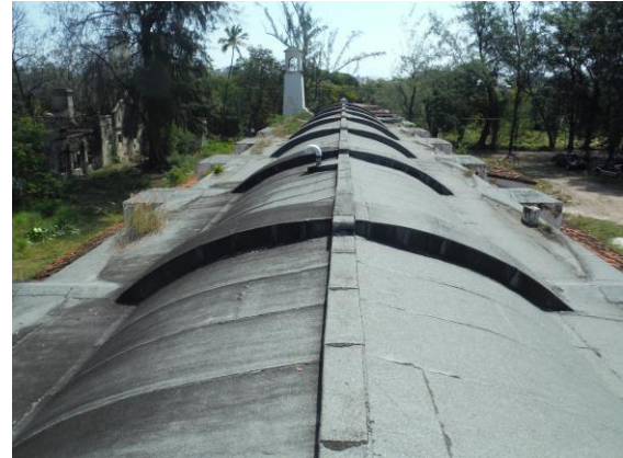
Figure 6 Barrel Vault Roof with Inverted Beam
