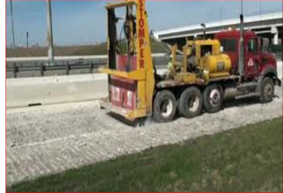
LL Engineering - The Stomper Demolition Guillotine Pavement
