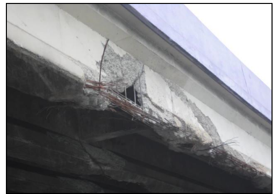
Figure 1 Bridge 897 - Cracking on Prestressed Concrete Girder Located P.R. 22 Eastbound Highway over P.R. 2 (Obtained from: Puerto Rico Highway and Transportation Authority)
