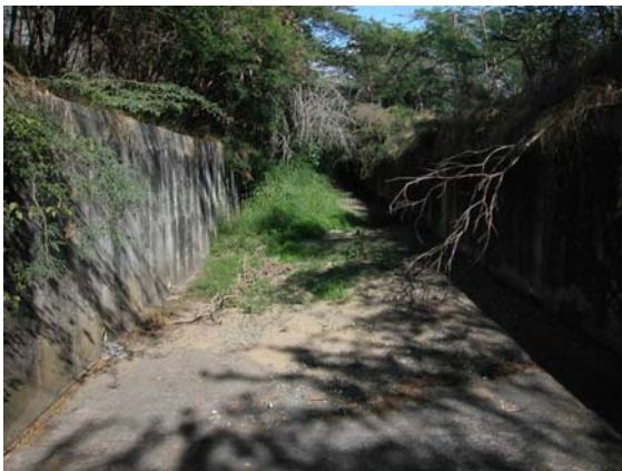
Figure 5 Concrete Streambank (Río Yauco, PR)
