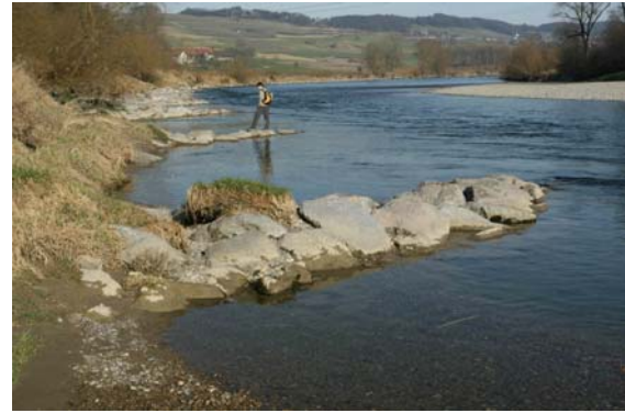
Figure 10 Rock Vanes used for Streambank Erosion Control
