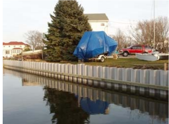
Figure 6 Sheet Piles used in Rivers
