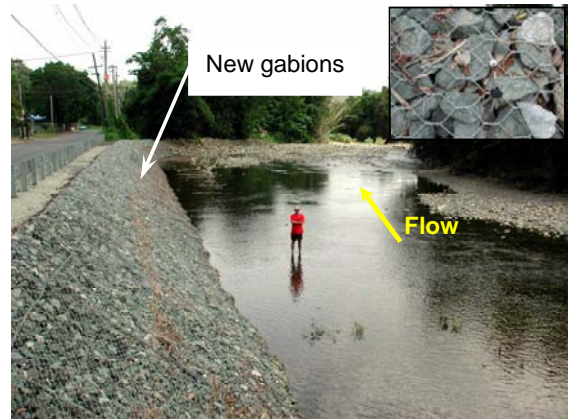
Figure 7 Río Mameyes, PR Newly Installed Gabions (2000)
