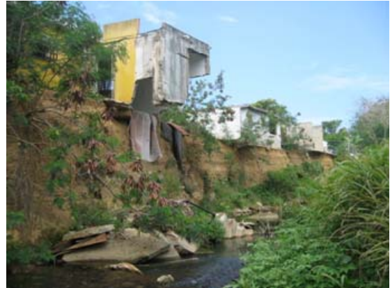
Figure 1 River Bank Eroded and Part of the Houses that Fallen into the River
